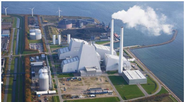
Ørsted's Avedøre Power Station in the Greater Copenhagen area. Credit: Ørsted.
